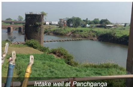
Intake well at Panchanga
